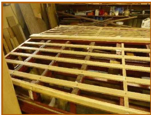
New battens attached to frames.
